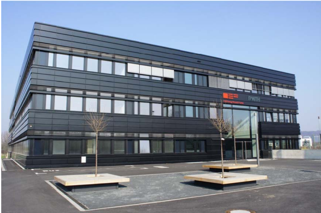
Figure 14: View of the E.ON ERC Main Building in Aachen, Germany
